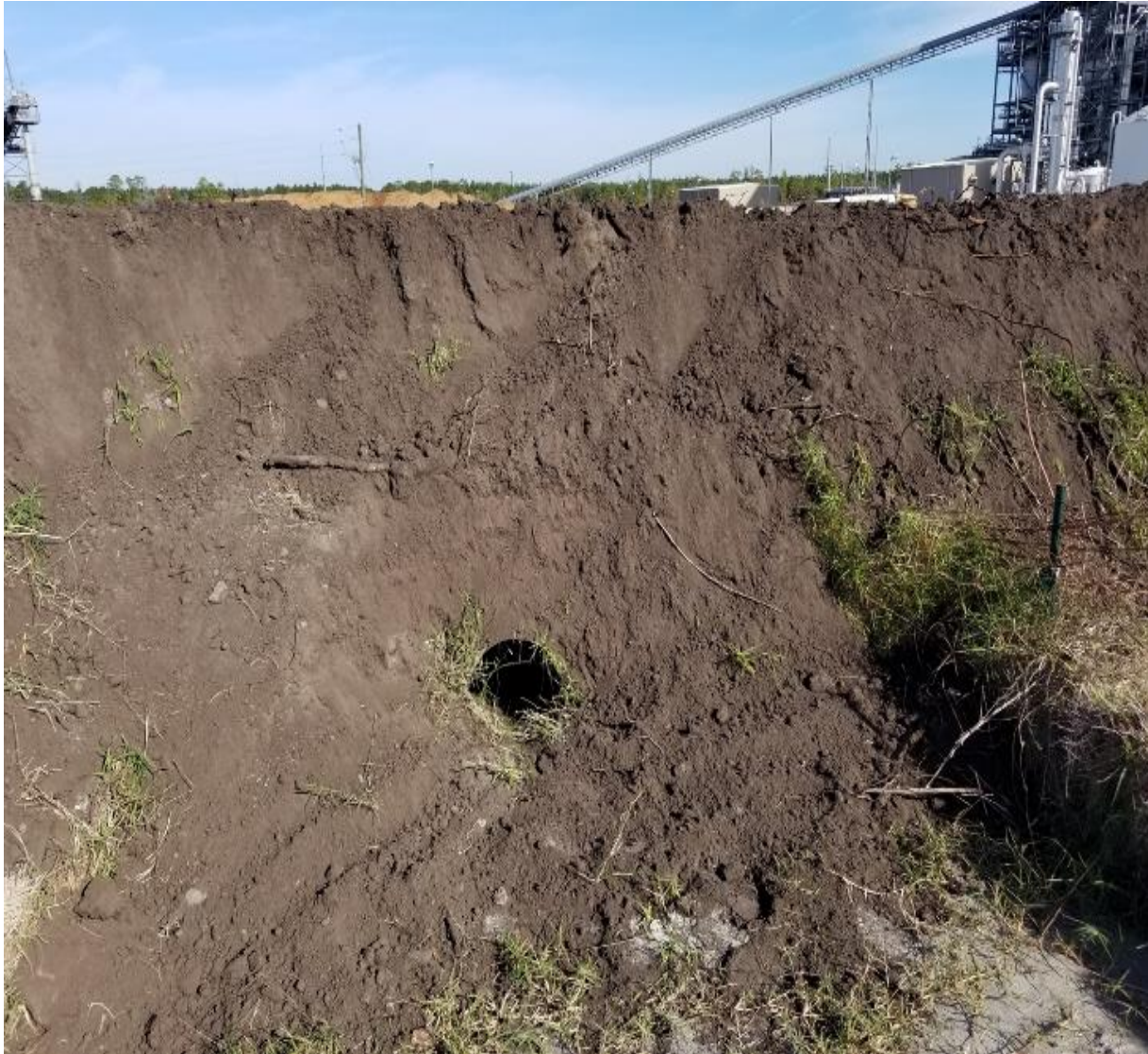
Figure 9. Cell 2 downcomer inlet surrounded by soil
